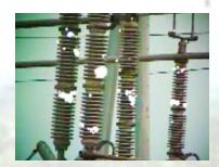
The pictures above show pictures from a substation with heavy Electrical Corona on most of the insulators and bushings. It was recorded with a DayCor® Solarblind Corona Camera where they had major problems with contamination.
